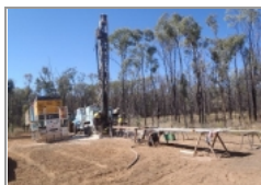
Drilling at Moorlands in central Queensland.
