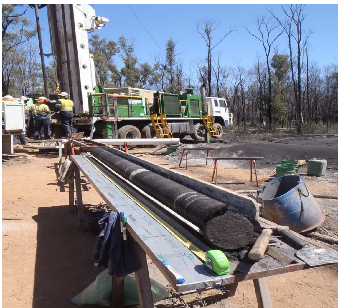
Photo of recent drilling activities conducted at Cuesta’s Moorlands Project
